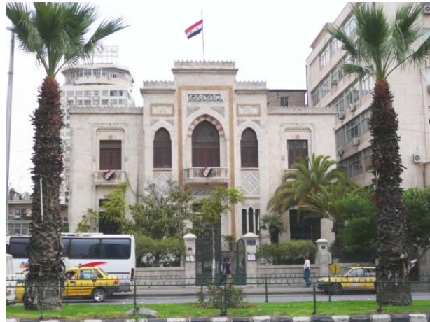
Figure 3. 'Abd al-Razzaq Malas, headquarters of the Fijeh water company, Damascus, 1937–1942. Photograph by the author.
